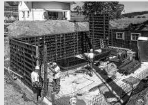
Wall Formwork
