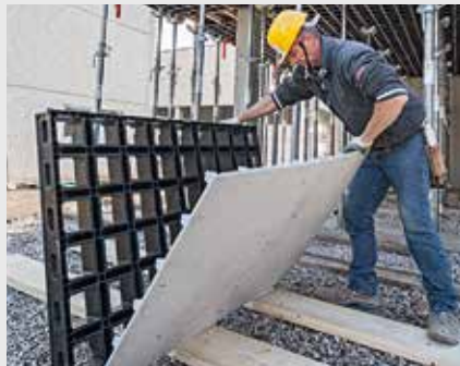
2. Removing the damaged formlining
