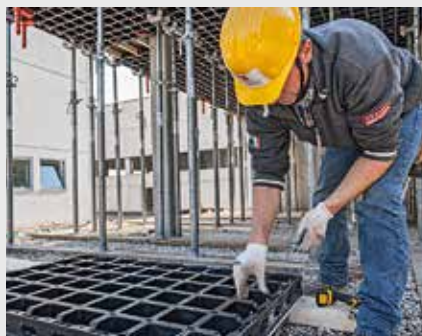
4. Screwing on the new formlining
