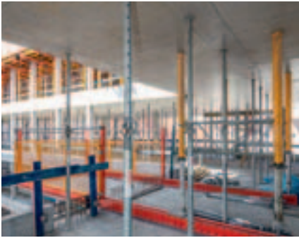
The RCS Rails of the RCS MP Landing Platform are clamped between two floor slabs by means of MULTIPROP Props.
