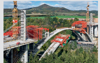
Bridge Formwork
