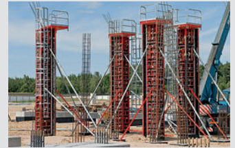
Column Formwork
